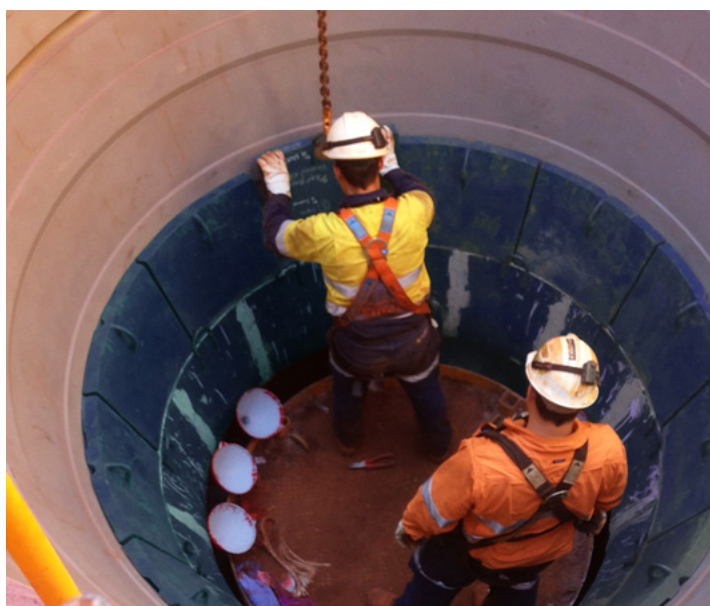
Concave liner installation
